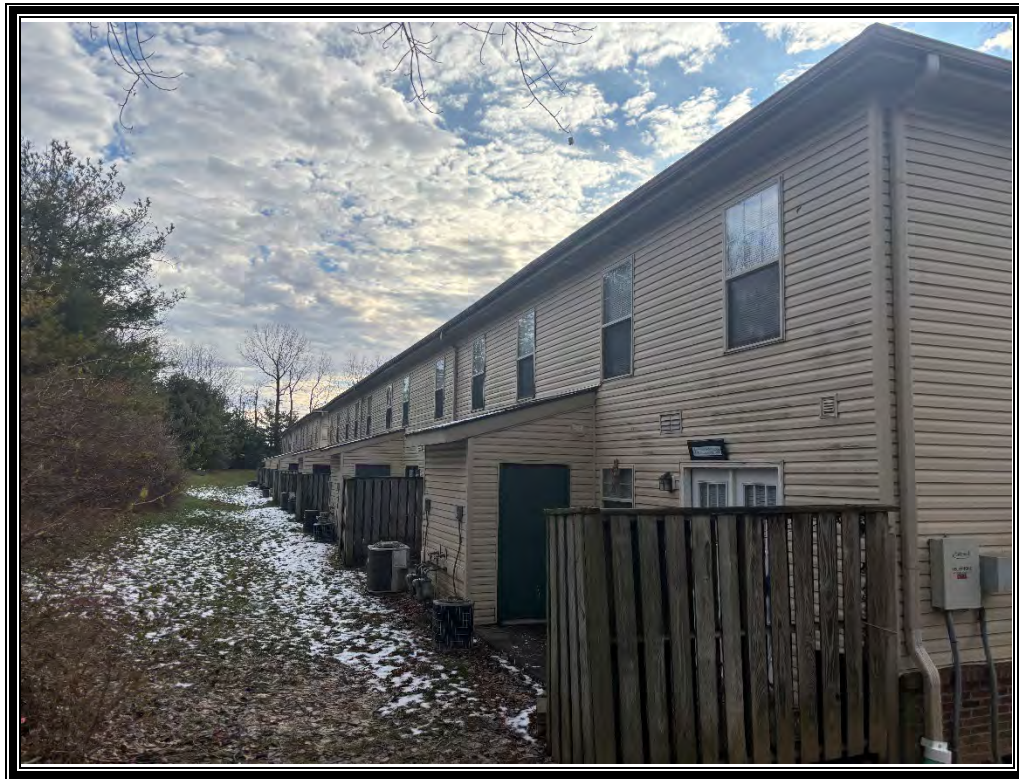
Photo 3: Representative view of the rear of an apartment building on the property.
