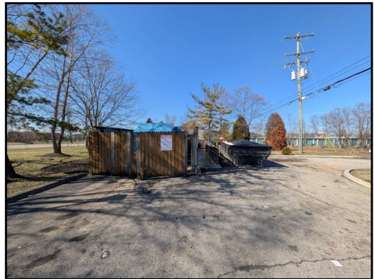
Photo 8 - Representative view of solid waste dumpsters/compactor
