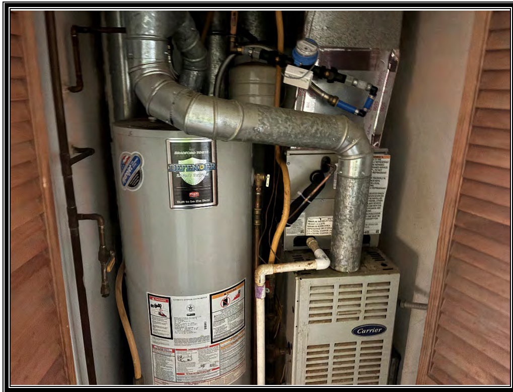
Photo 11: Representative view of a unit's utility closet on the property.
