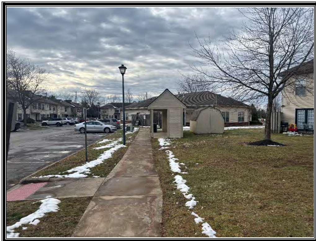
Photo 4: View of the mailbox structure and shed located near the leasing office.
