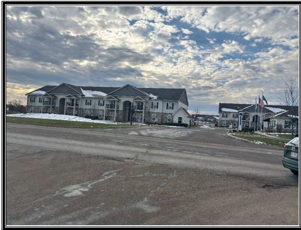
Photo 13: View of the south adjoining multi-family residential complex.
