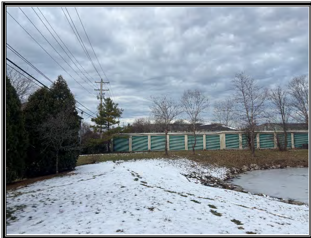
Photo 14: View of the west adjoining self-storage facility.
