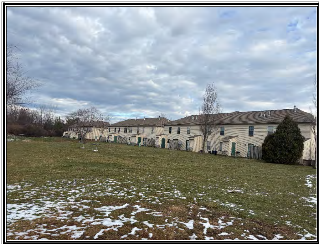
Photo 2: Northerly view of apartment buildings on the western portion of the property.
