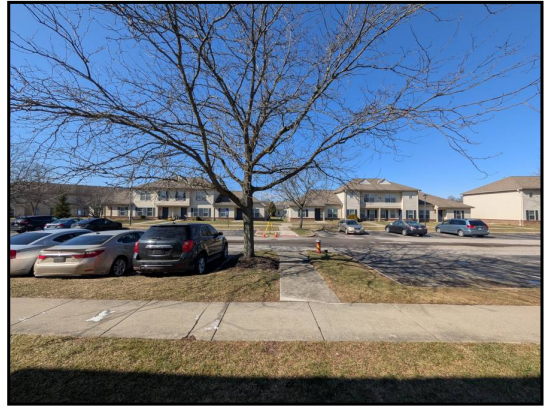
Photo 18 - View from the east boundary, looking west
