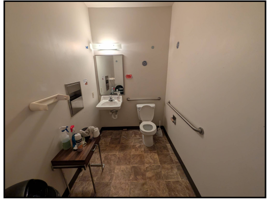
Photo 22 - Typical view of the leasing office restrooms
